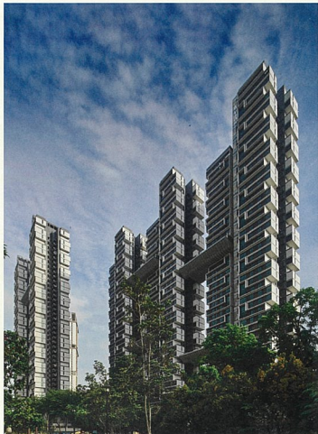
Order as Clarity — As an efficient and economical baseline of architecture, the orthogonal box carries an inherent structural logic. We can achieve further order and clarity by organizing them into geometric groups. Skyterrace@Dawson, Singapore
